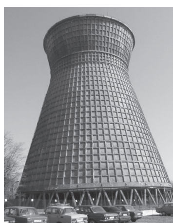
III. 4. Iron concrete prefabricated cooling tower station #4 Darnytsia Combined heat and Power Plant in Kyiv City
