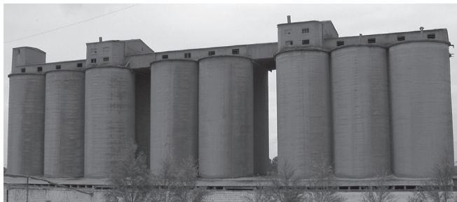
Ill. 6. Iron concrete monolithic silages of the building #6 Open Joint Stock Company 'Mykolaiv Cement'
