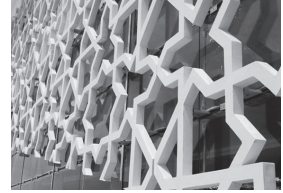
III. 12. Application of RPC (Reactive Powder Concrete) – “Ductal®”: façade panels – sun-shades (“double-skin façade”=“building envelope”), a – Plescop City Hall, Plescop, France, 2010, b – Rabat-Salé Airport building, Rabat, Morocco, 2011 [52]
