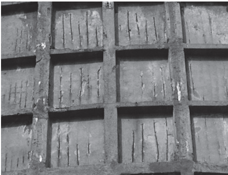
Ill. 11. Steel reinforcement corrosion and destruction of concrete of upper belt of firmness of the cooling tower #4 at Darnytsia Combined heat and Power Plant, protective layer of concrete is lower than designed
