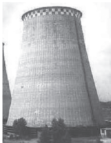
III. 2. Iron concrete monolithic cooling tower station #1 Kyiv Combined heat and Power Plant-6
