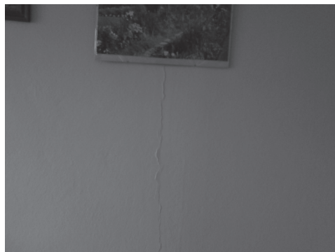
Ill. 6b. System joint – leak in place of vertical joint in building number 1
