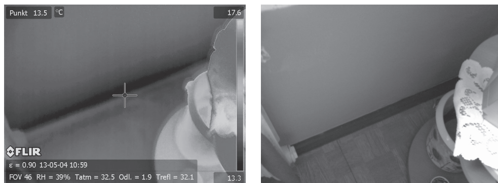
Ill. 7. Thermal bridge – connection between floor and external wall in building number 1
