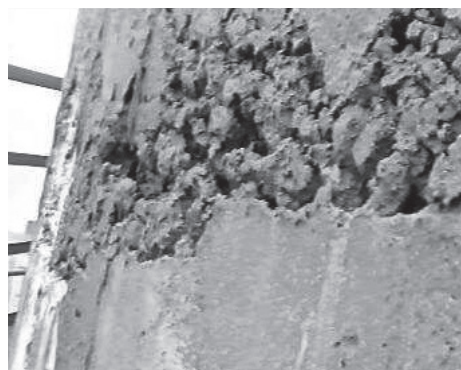
Ill. 13. Insufficiently compressed concrete at the joint of tier of concreting
