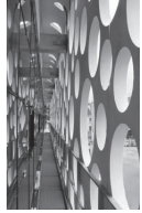
III. 12. Application of RPC (Reactive Powder Concrete) – “Ductal®”: façade panels – sun-shades (“double-skin façade”=“building envelope”), a – Plescop City Hall, Plescop, France, 2010, b – Rabat-Salé Airport building, Rabat, Morocco, 2011 [52]
