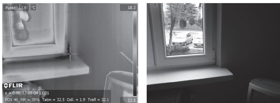
Ill. 8. Thermal bridge – connection between window jamb and external wall in building number 1
