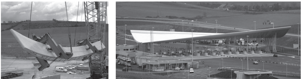
III. 8. Application of RPC (Reactive Powder Concrete) – “BSI/CERACEM®”: shed: Millau Viaduct Toll Gate, Millau, France, 2004 [49, 56]
