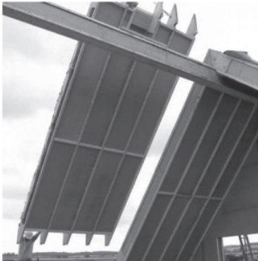
III. 8. Assembly of plate elements [10]
