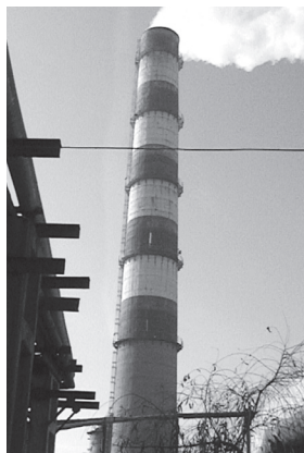
Ill. 5. Iron concrete monolithic pipe H = 120 m Kyiv Station #2
