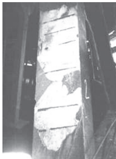
Ill. 8. Insufficient thickness of protective concrete layer and corrosion of transversal reinforcement in the pillar of leaning colonnade of cooling tower station #1 Kyiv Combined heat and Power Plant 6
