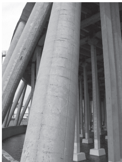
Ill. 7. The lengthwise and cross-cut cracks in pillars of leaning colonnade of cooling tower station #5 of Rivne Power Station
