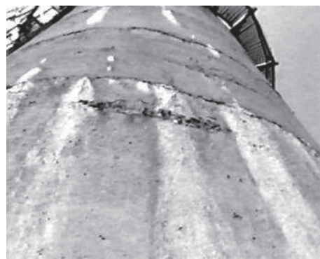
Ill. 14. Sulfate corrosion of concrete, filtration of moisture at the joint of concreting
